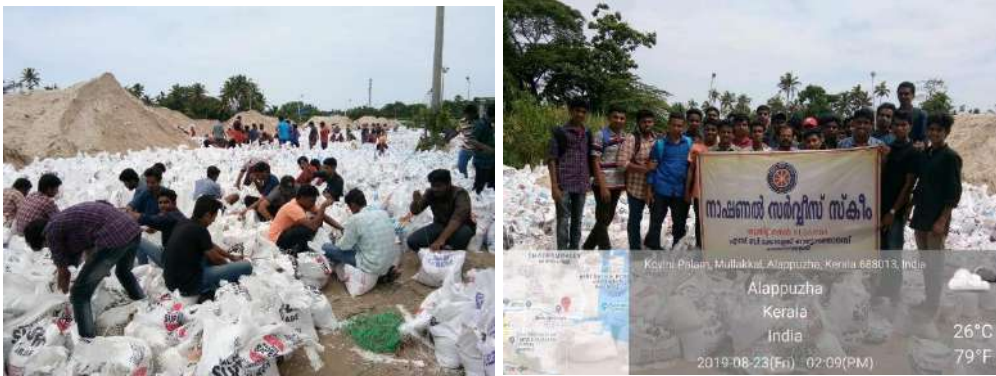
(NSS Volunteers helping in the construction of bund in Mullakkal, Alappuzha)
